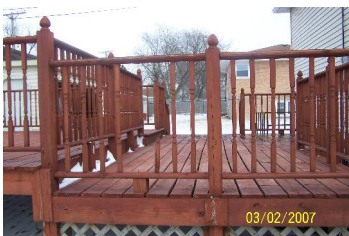
06-1. Decks/Porch SAMPLE PICTURES
