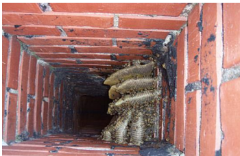
11-1. Chimney(s) SAMPLE PICTURES
