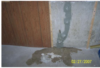
18a-1. Basement SAMPLE PICTURES
